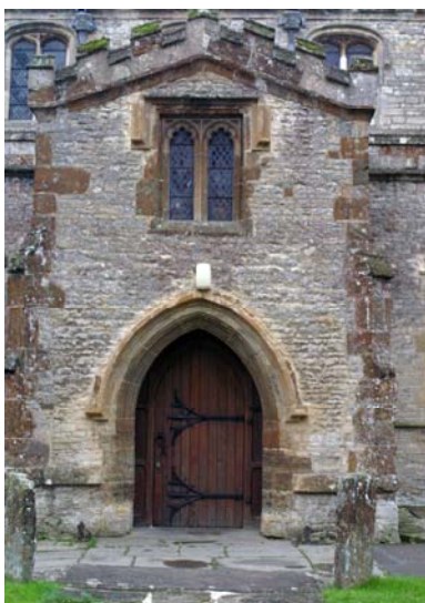
St. Egburg's Church is the oldest building in Bicester and is a few minutes walk from the hotel. It has been here for 900 years.
